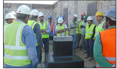
Demonstration of Structural Waterproofing
