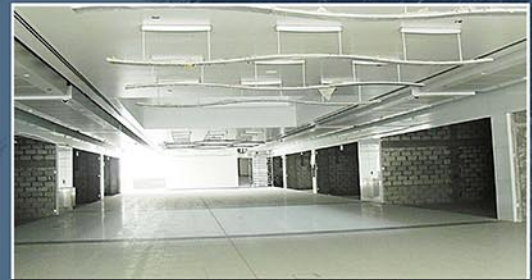
Barwa Commercial Avenue Building Project Site
