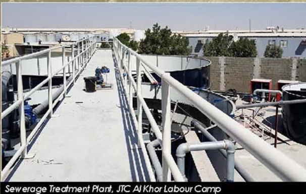
Sewerage Treatment Plant, JTC Al Khor Labour Camp
