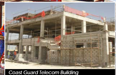
Coast Guard Telecom Building
