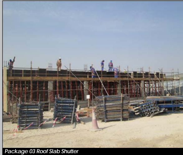
Package 03 Roof Slab Shutter
