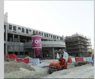
Ahmad Bin Hanbal Secondary School Engr. Mohammed Abu Deeb (Site Manager)
